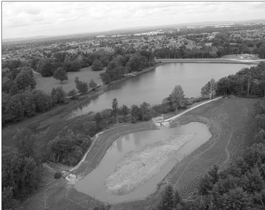
Figure 9. Borrow area at Tilgate (before planting)
