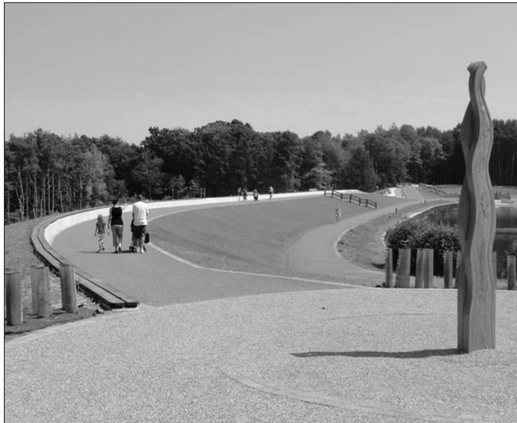
Figure 8. View of completed crest at Tilgate, including seating on rear crest wall
